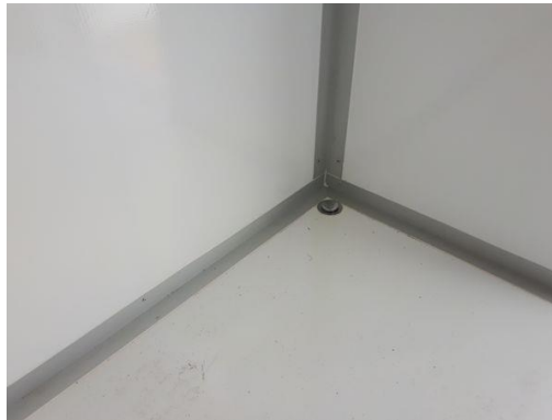
Figure 1: Sample photo of a drain plug installed
