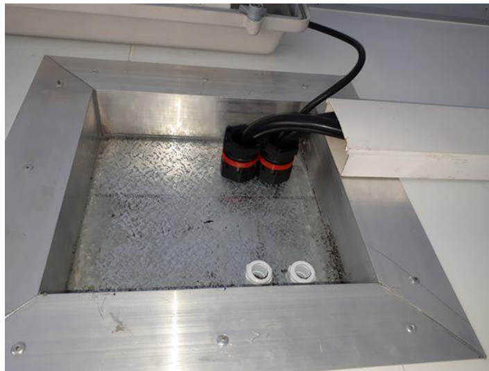
Figure 9: Battery room gland plate
