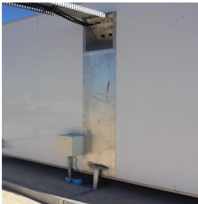
Figure 2: Aluminium plate and earth connection points
