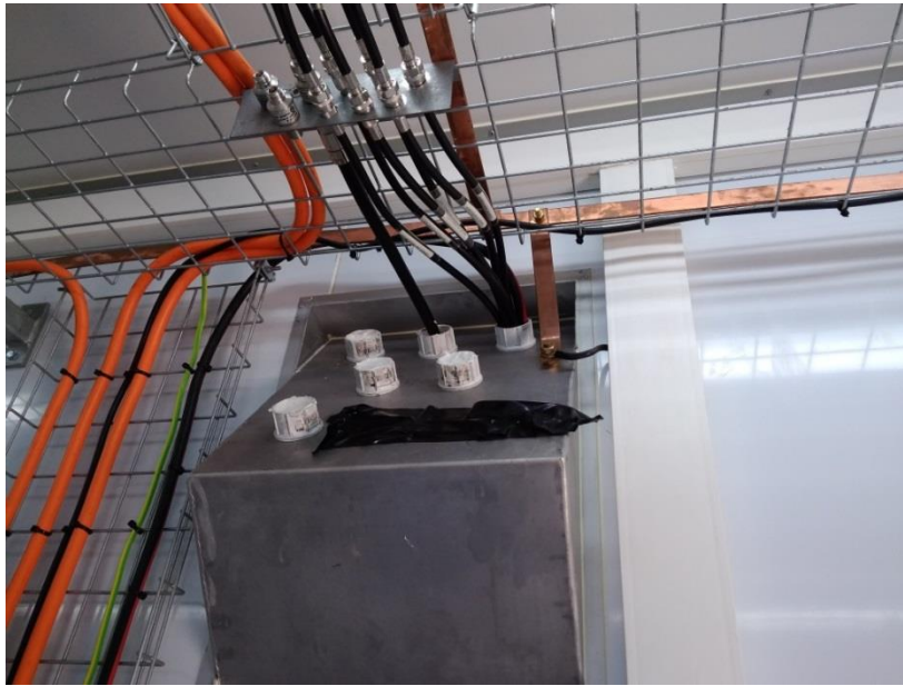
Figure 7: Mounting plate for RF lightning surge protectors
