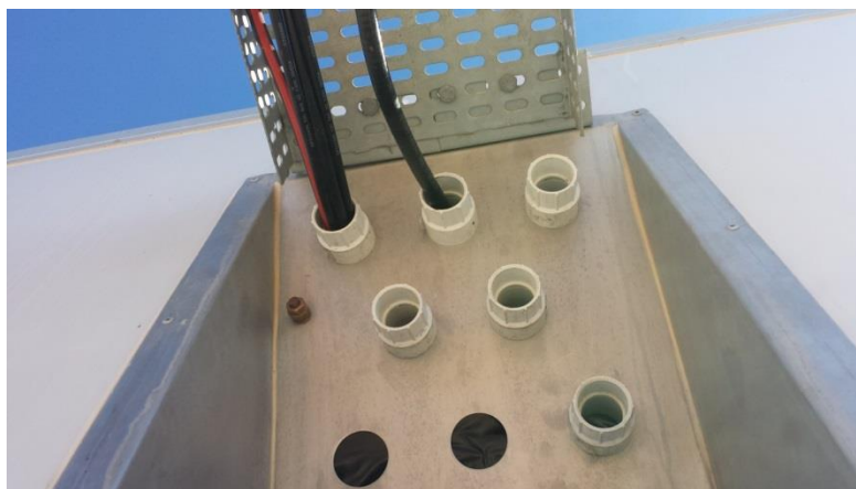
Figure 6: Feeder entry panel
